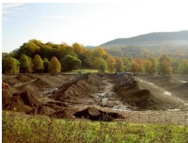
Maya Lin, Storm King Wavefield, 2007–08 (construction view I, 2007). Image Credit: Katie Commodore, Courtesy Storm King Art Center Archives
